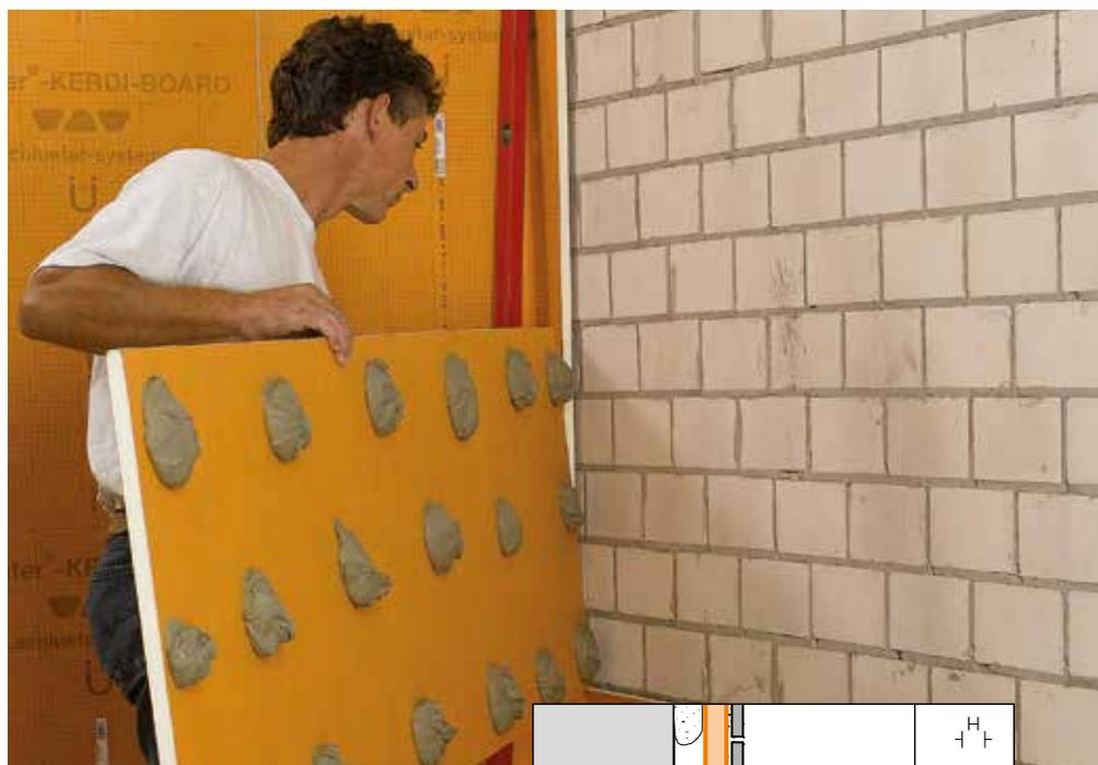
suitable adhesive or mortar. If necessary, the material may be secured with additional wall anchors. In the case of stud frames made of wood or metal, Schlüter®-KERDI-BOARD is attached with screws from the matching hardware system.
