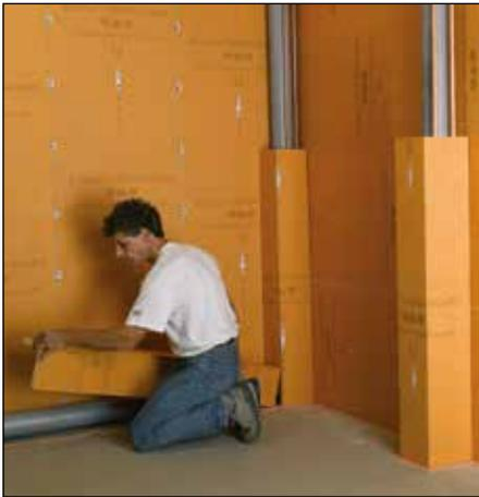
**Note:** See section “Waterproofing” on the use of Schlüter®-KERDI-BOARD in bonded waterproofing assemblies.
